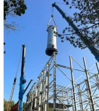
Figure 18-2. Installation of the main vessel of th ATHENA facility. Photo provided by Ilie Turcu.
