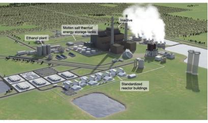
Figure 2-4. Rendering of a repowered 1,200-MWe two-steam-unit plant (2.24). Graphic from Terra Praxis, 2022.
