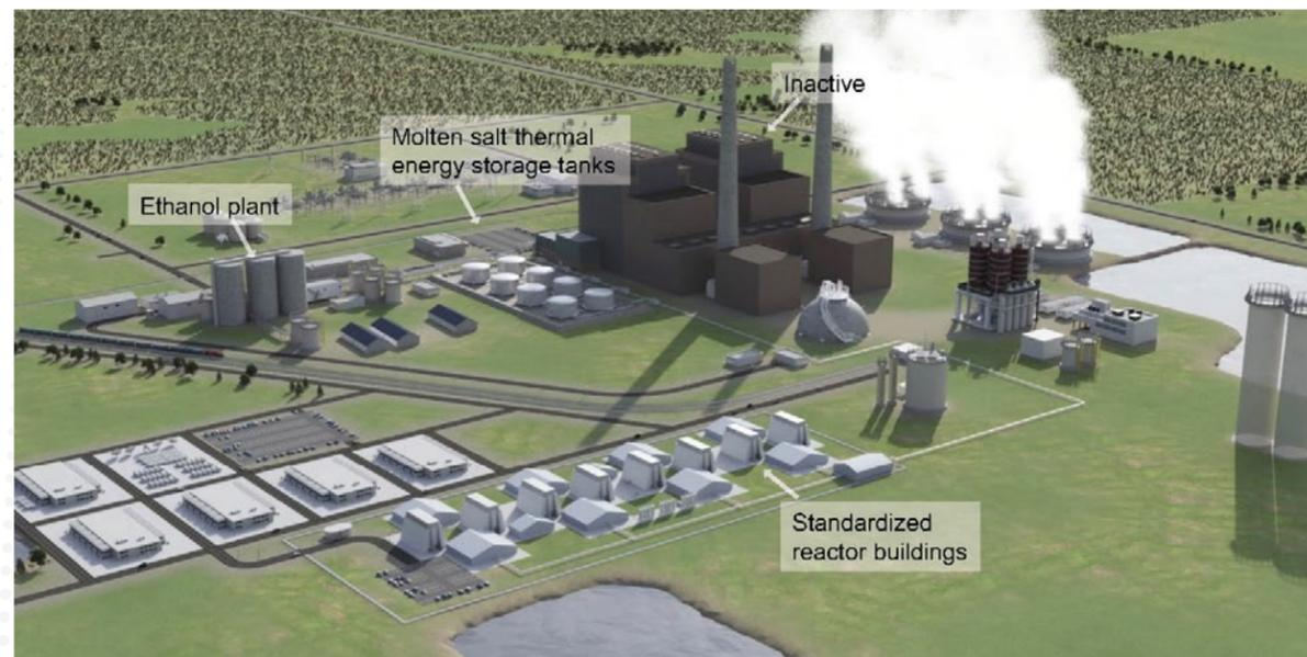
Figure 14- 3. Rendering of a repowered 1,200-MWe, two-steam-unit plant (14.9).
