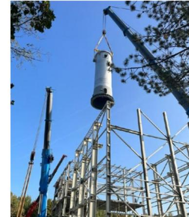
Figure 18-2. Installation of the main vessel of the ATHENA facility. Photo provided by Ilie Turcu.
