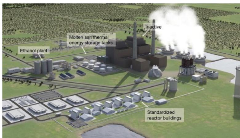
Figure 15- 1. Repowering coal case study: two-steam-unit, 1,200-MWe plant (15.5)
