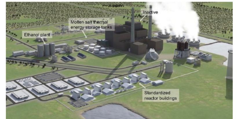
Figure 12- 1. Repowering coal case study of Coal Creek Station, conceptual repowering of a two-steam-unit, 1,200-MW electric plant with eight advanced reactors and thermal storage (turbine halls and storage units in the foreground). Image credit: Terra Praxis.
