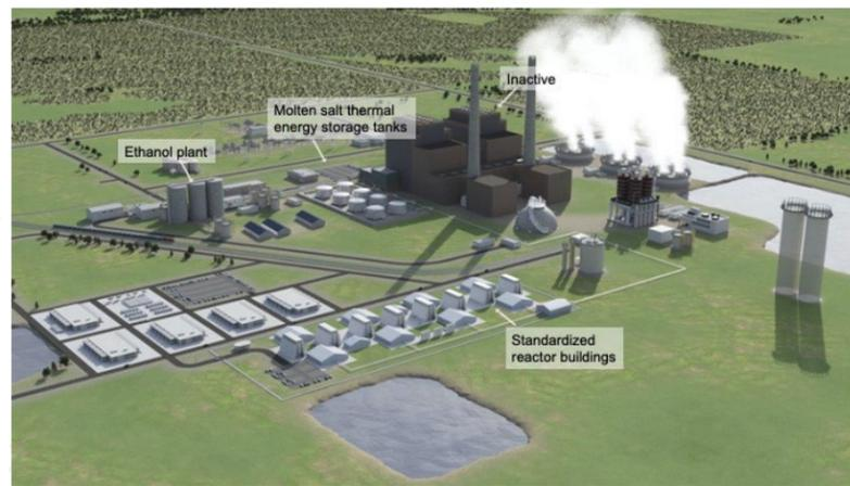
Figure 2- 4. Rendering of a repowered 1,200-MWe two-steam-unit plant (2.24). Graphic from Terra Praxis, 2022.
