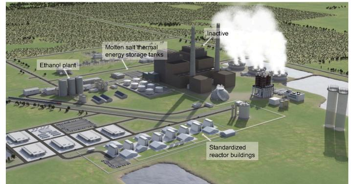
Figure 1. Repowering coal case study: two-steam-unit, 1,200 MWe plant<sup>5</sup>
